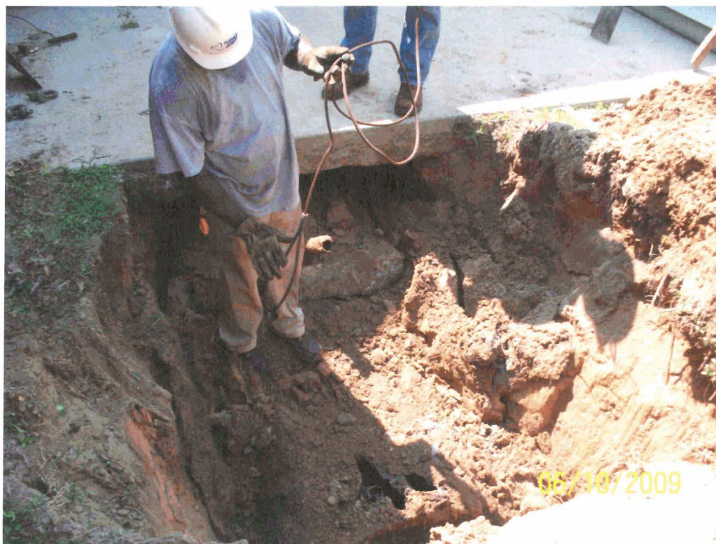
Picture 2: UST 1064Gardenia during excavation and removal.
